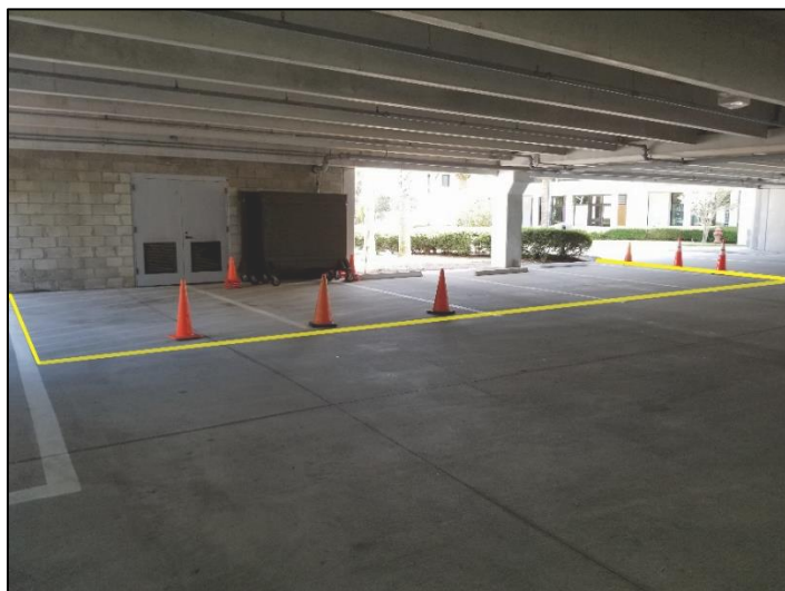
Designated solicitation and political signage area located immediately on the right as you enter the parking garage.
